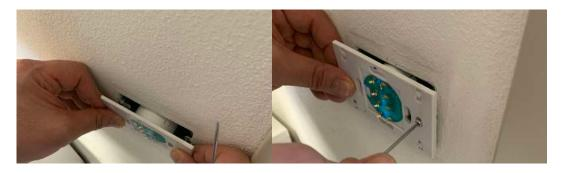
[5] Check all KNX functions before to install front panel.
