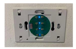
If KNX works well without front panel it means that hardware is OK.
